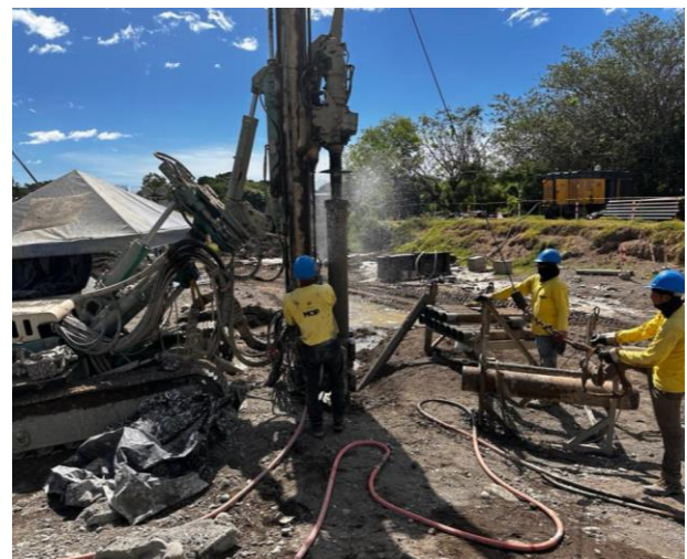
Figure 3. Perforation of one testing micropile
